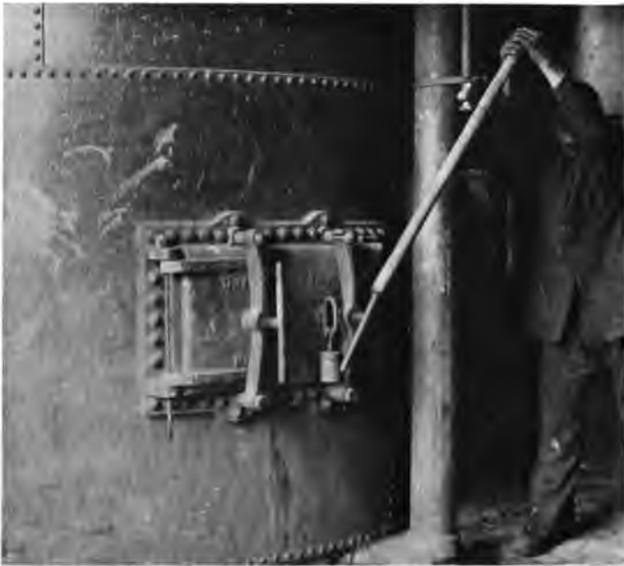
Fig. 1. Dangerous Method of Tightening Cotter Bars.*
